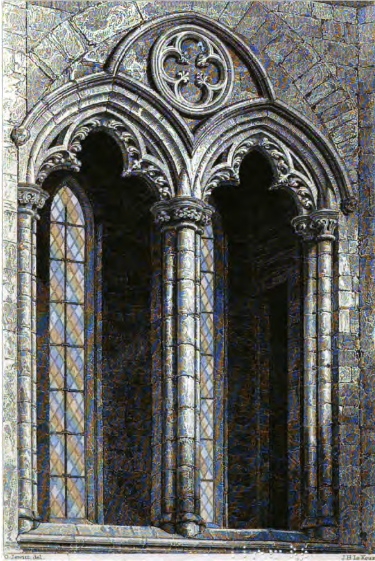
WEST WINDOW OF RAUNDS CHURCH. [RESTORED]
